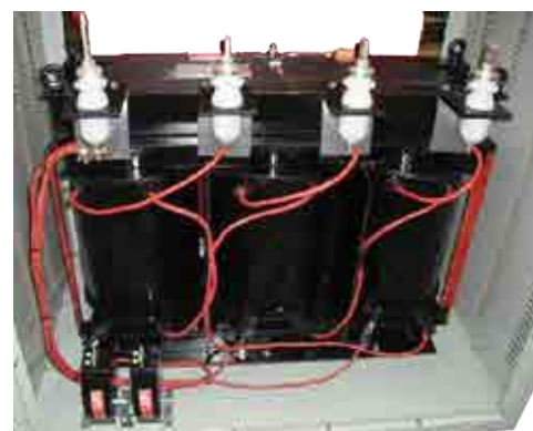
THREE PHASE ENCLOSED TYPE NEUTRAL EARTHING TRANSFORMER (ZIG-ZAG) COMPLETE WITH HV BUSHING AND CT
